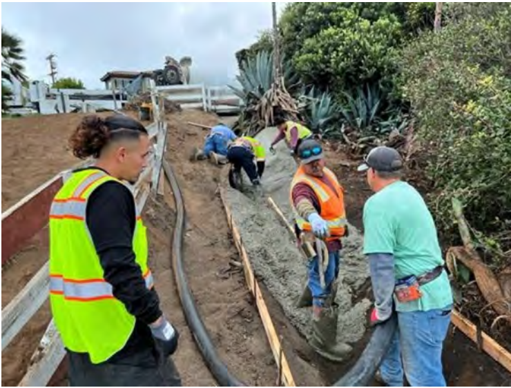
San Diego city crews work on repairs to a storm drain at La Jolla Hermosa Park in Bird Rock. (San Diego Stormwater Department)
